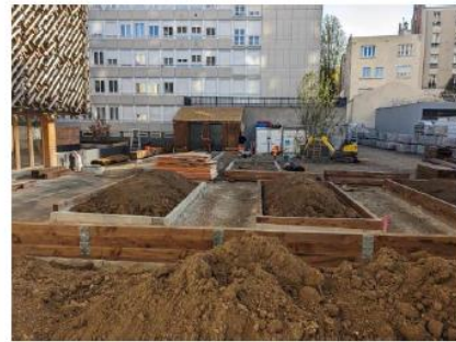
Shared garden's installation
